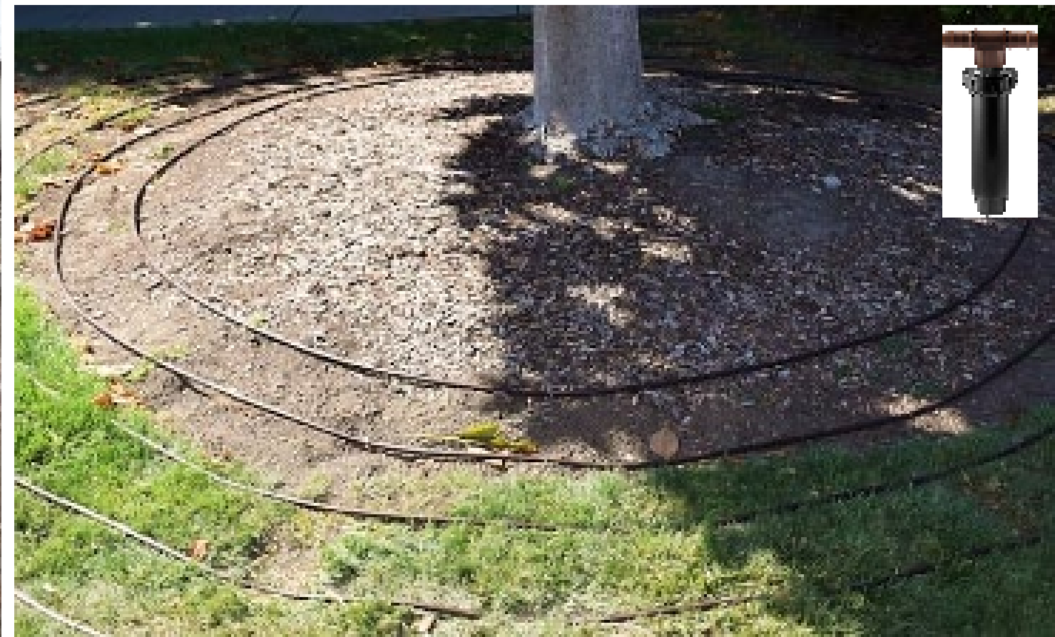
5 Drip rings (500' of 6gph -12x18) at dripline– 30' dia canopy Spray to Drip Retrofit Kits – up to 360 GPH ea
