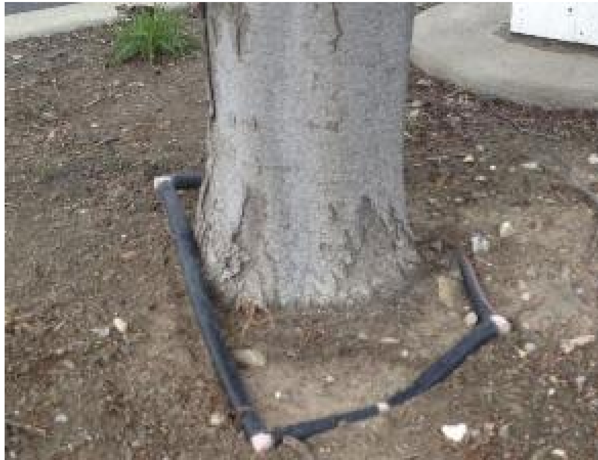
Insufficient tubing on mature tree and too close to flare
