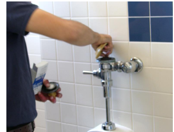
Source: Valley Water, flush-valve diaphragm being retrofitted
