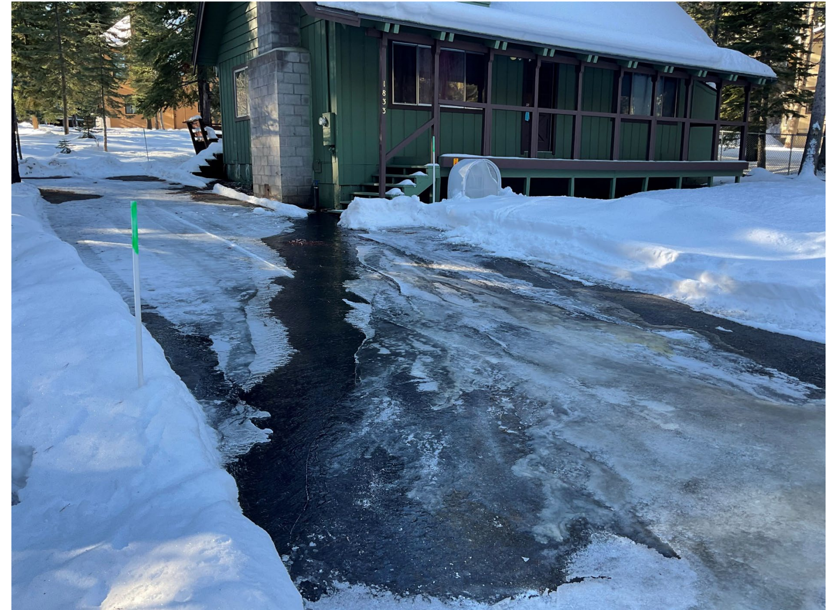
Burst pipe caught with AMI data
