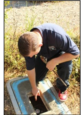
An auditor uses the meter to check for leaks.
