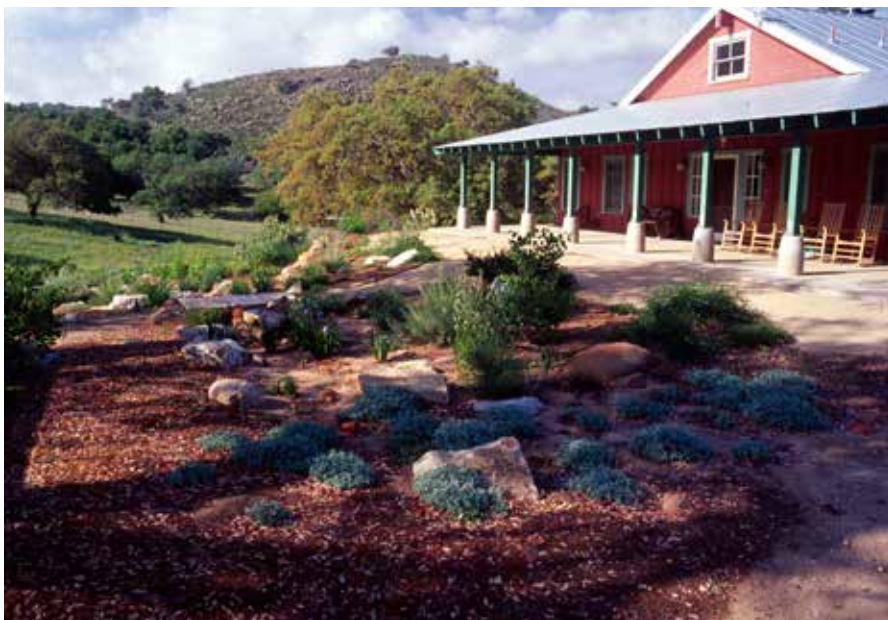
Figure 2: The 8 foot decomposed granite apron around this house has helped it withstand two major fire events in 2003 and 2007.
