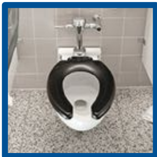
Flushometer Valve Toilets
