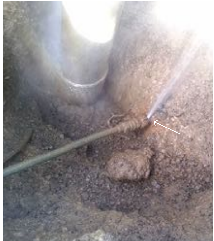
Leak on 1" corporation stop; replaced corp. stop and lateral
