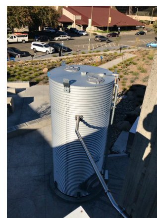
Images clockwise (top) City of Santa Rosa City Hall Sustainable Education Garden, post installation of the turf conversion and low impact development project. Features include CA native and low water use plants, swales, bio-retention, drip irrigation and weather-based irrigation amongst others; (bottom right) 1,200 gallon rainwater harvesting tank on display in outdoor classroom and gathering area; (bottom left) swale capturing, cleaning and infiltrating stormwater runoff. Source: City of Santa Rosa
