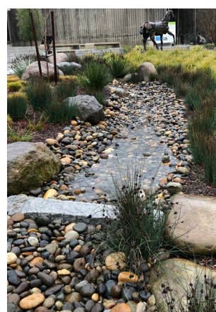
Images clockwise (top) City of Santa Rosa City Hall Sustainable Education Garden, post installation of the turf conversion and low impact development project. Features include CA native and low water use plants, swales, bio-retention, drip irrigation and weather-based irrigation amongst others; (bottom right) 1,200 gallon rainwater harvesting tank on display in outdoor classroom and gathering area; (bottom left) swale capturing, cleaning and infiltrating stormwater runoff. Source: City of Santa Rosa
